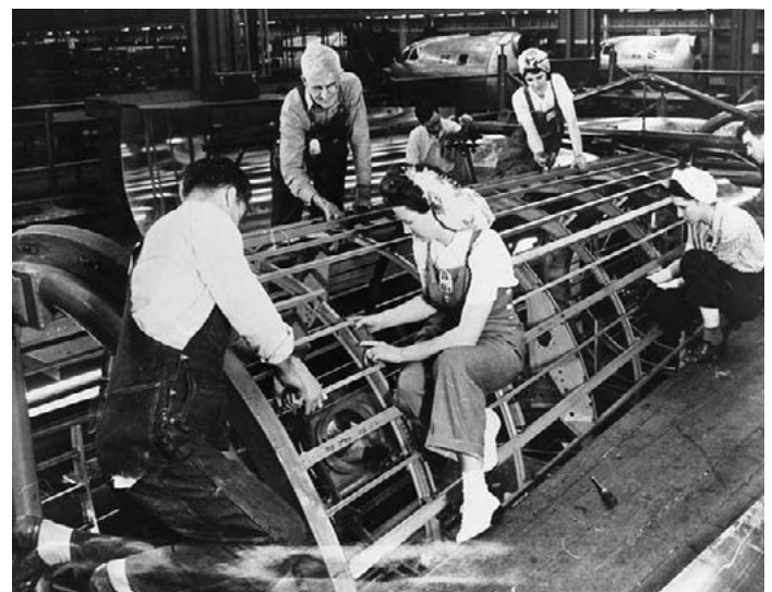
ABOVE Bell Bomber Plant Employees Working on the Fuselage of a B-29 Bomber Unidentified photographer, 1943-1945 Gift of Lockheed Aircraft Corporation, 1952
