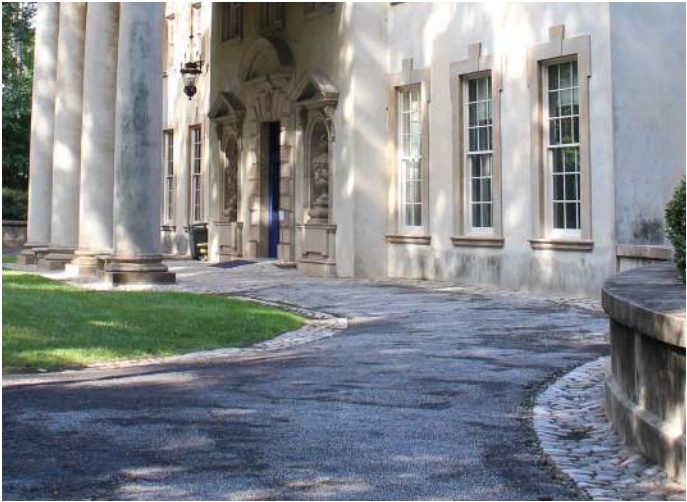
FAR TOP The new Swan House driveway is made from a special concrete mix containing granite fines. TOP Asphalt installed in the 1960s needed to be replaced.
