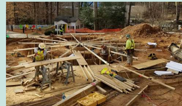
Olguita's Garden, water feature under construction. Photograph by Sarah Roberts.
